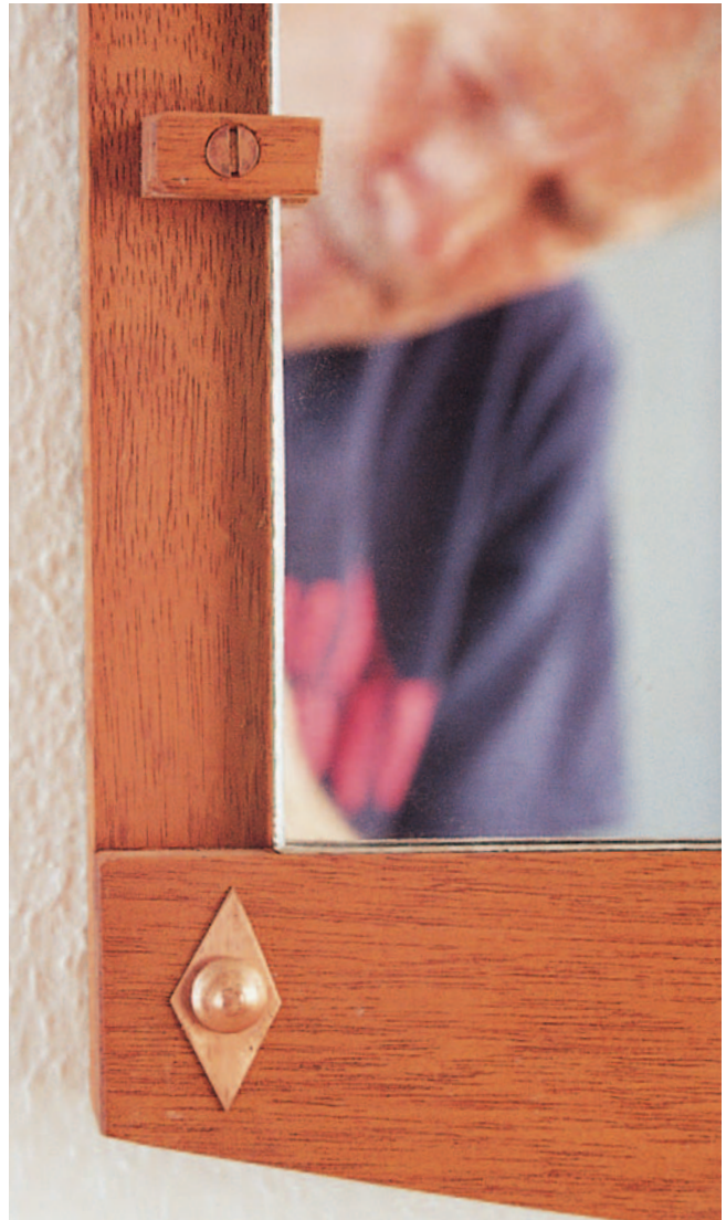
The author used lap-jointed corners secured with copper nails and set off by decorative copper diamonds, materials he had on hand.
